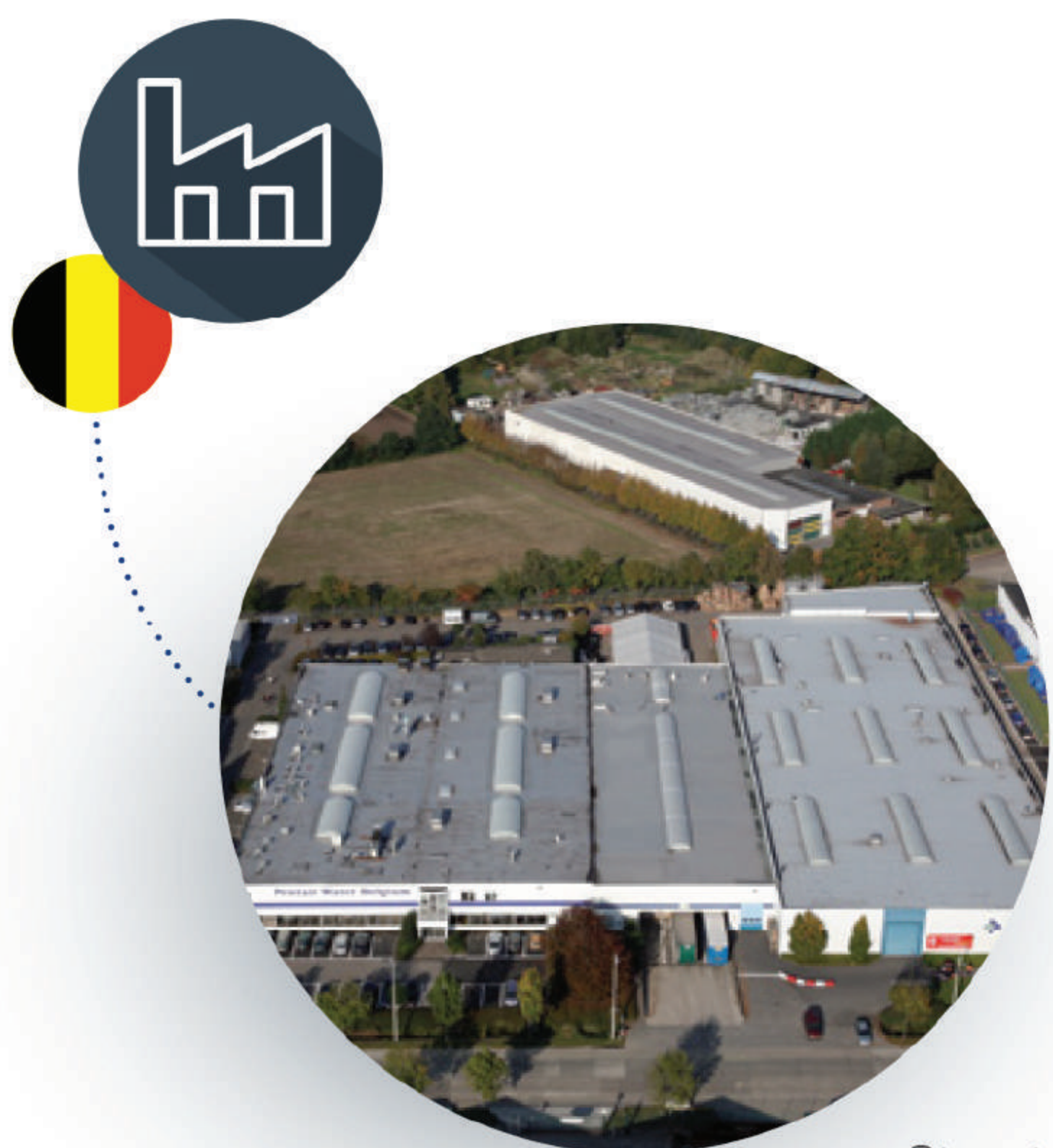
Structural production site Herentals, Belgium
