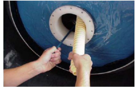
Step 3: Put assembly inside the tank to mount laterals.
